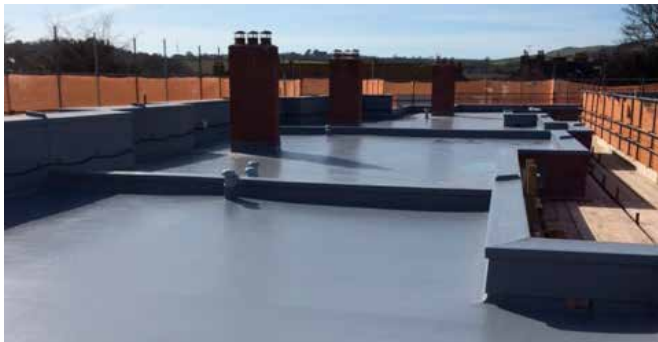
1200m 2 - Housing Association roof
