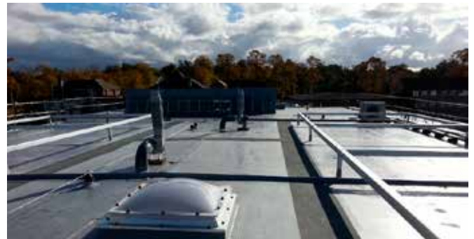
800m 2 - High School roof
