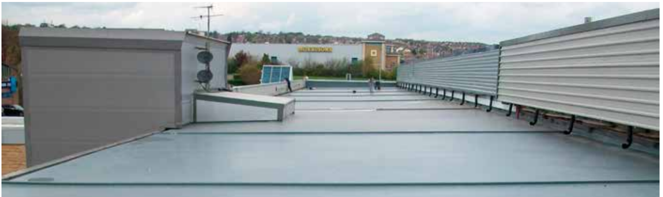
1000m 2 - Factory roof
